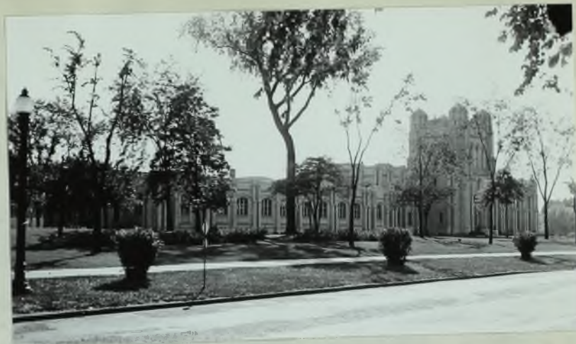
Figure 20. The new water filtration plant completed at Saginaw in 1930 supplies an abundance of pure water to all parts of the city.
