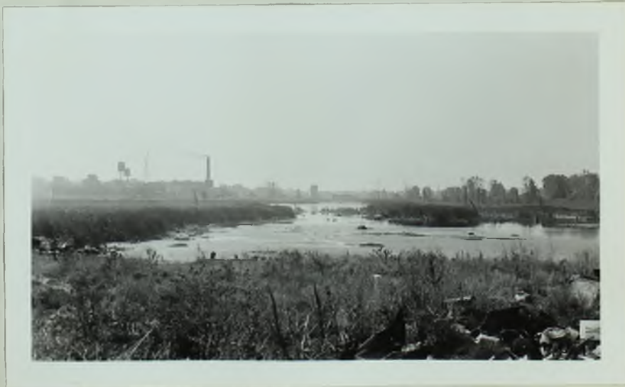
Figure 32. Low, swampy land such as that shown in this picture, is found in the northern part of Saginaw. The buildings seen in the distance are plants of the Chevrolet Motor Car Company.
