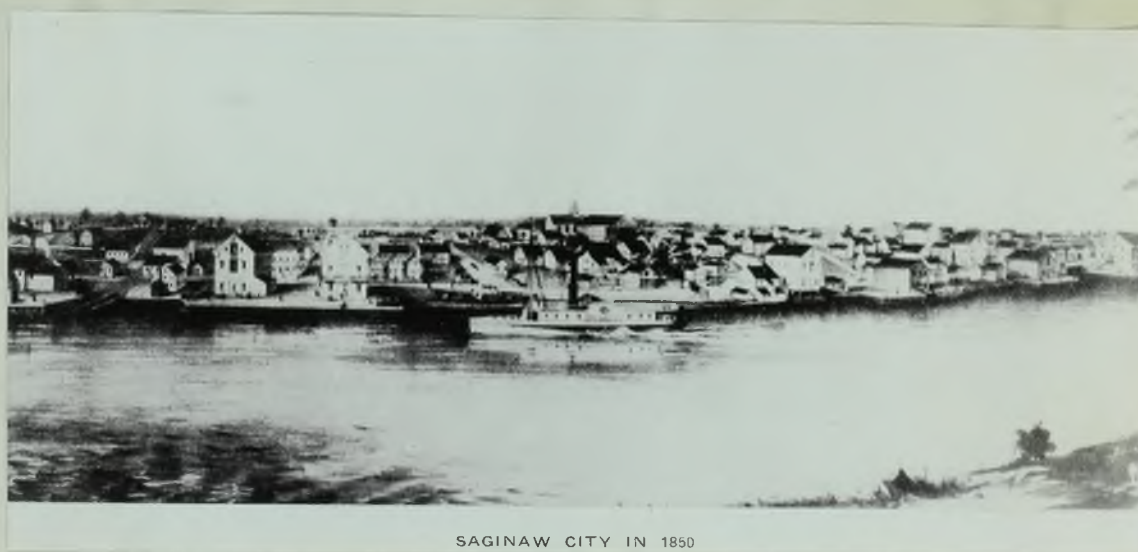
Figure 13. This early view of West Saginaw shows the abrupt rise of ground and high level land upon which much of the city was built. Docks and saw mills like those in the picture lined both sides of the river at Saginaw.—J.C.Mills' History of Saginaw County, Michigan , Vol. I, p.175.
