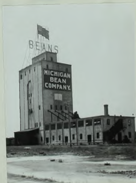
Figure 21. The largest beam elevator in the world is located at Saginaw.
